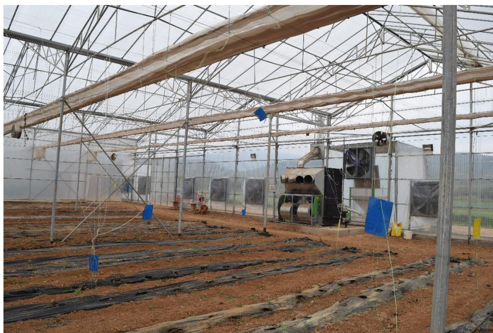
Figure 6: Hot air generator using agrobiomass at BOKARPOS Greenhouse (Source: PelleTech / Camino Design).
