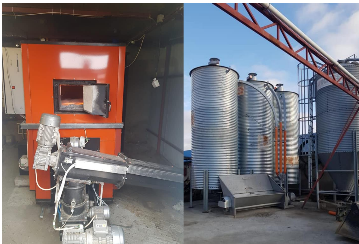
Figure 13: Agrobiomass boiler (150 kW) and silos for sunflower husks at Avicol Prod Consult Ltd. (Source: Biosistem).
