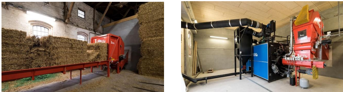
Figure 5: The straw feeding line (left) and the 800 kW straw boiler (right) at Orupgaard Estate (Source: Linka Energy A/S).
