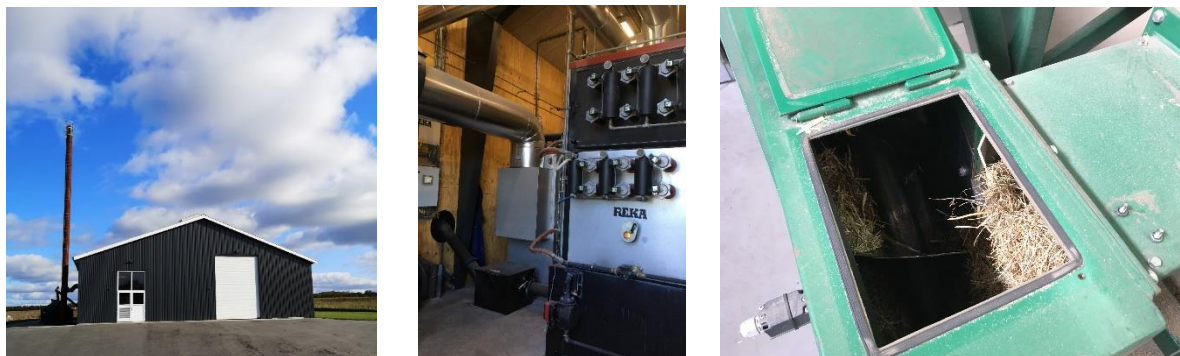
Figure 4: The straw-fired district heating plant at Ulbjerg (left), the straw boiler (middle) and close-up of the straw bale cutter (left) (Source: Kirsten Krogh and Louise Krogh Johnson).
