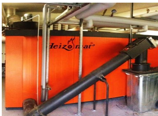
Figure 9: Retirement home at Chevresis and Heizomat biomass boiler installed (Source: Agronergy).
