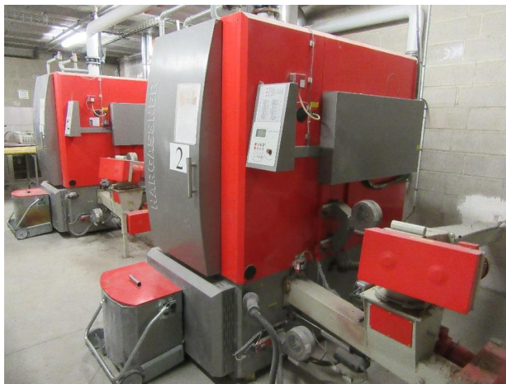
Figure 11: The ESAT ADAPEI 80 facility for social and professional integration of adults with disabilities located near Allaines (left) and the twin Hargassner biomass boilers fuelled with miscanthus (right) (Source: AILE).
