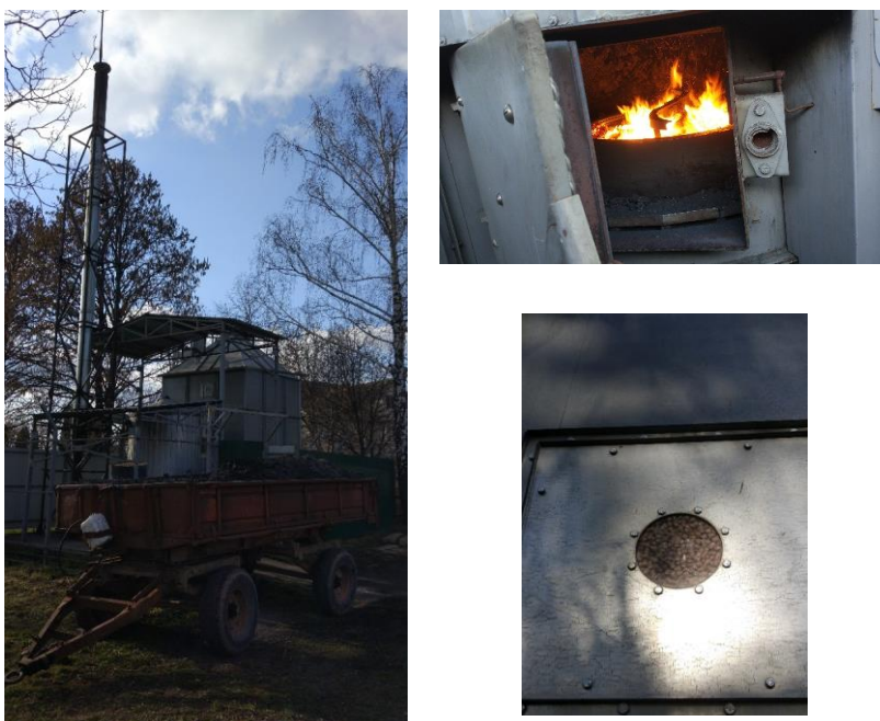
Figure 17: The AVERS straw pellet-fired boiler at Uman School #9 (Source: UABIO).
